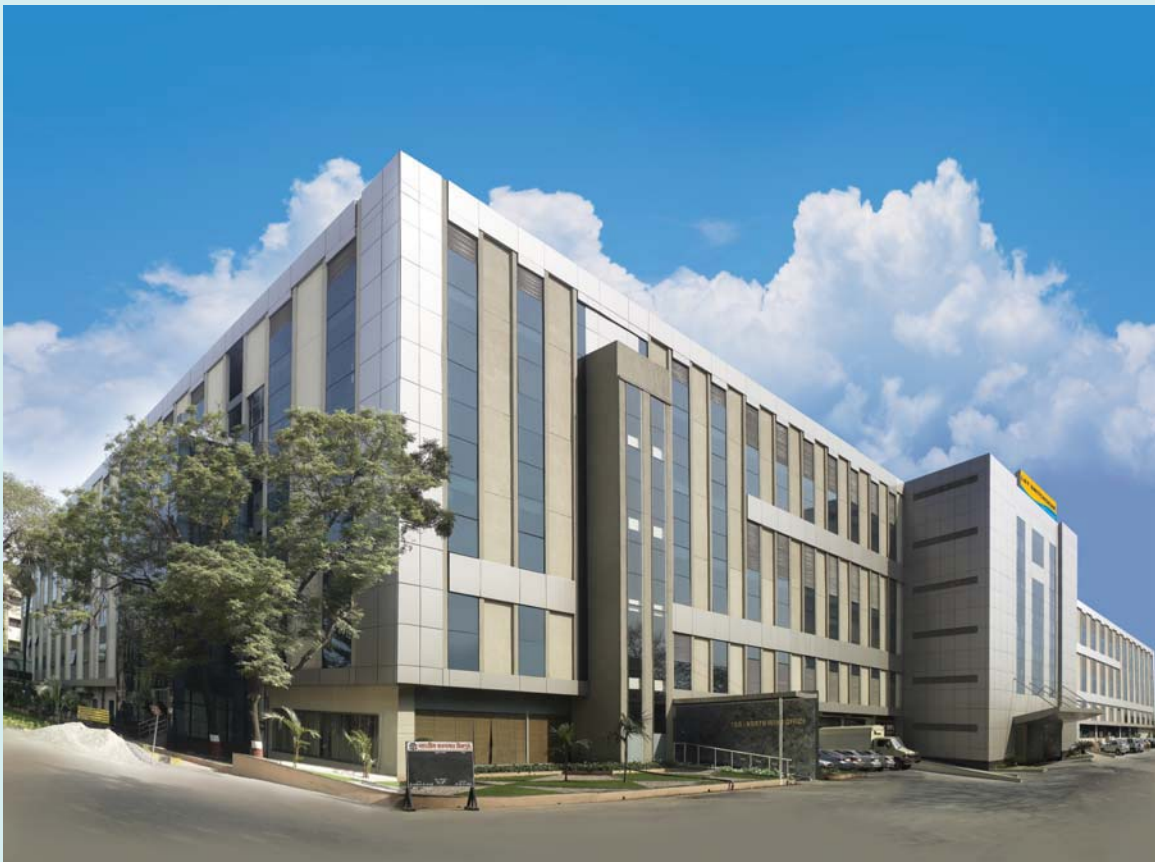
Switchgear Factory, Mumbai
