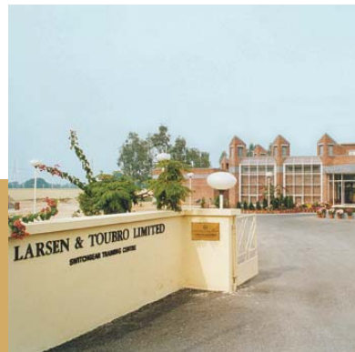
Switchgear Training Center, Lucknow
