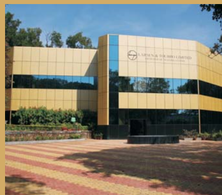
Switchgear Training Center, Pune
