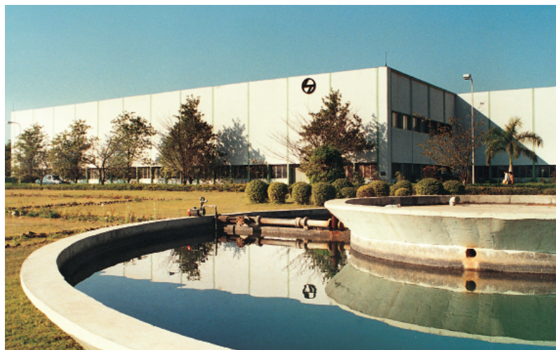
Switchgear Factory, Ahmednagar
