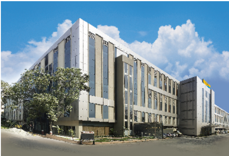
Switchgear Factory, Mumbai
