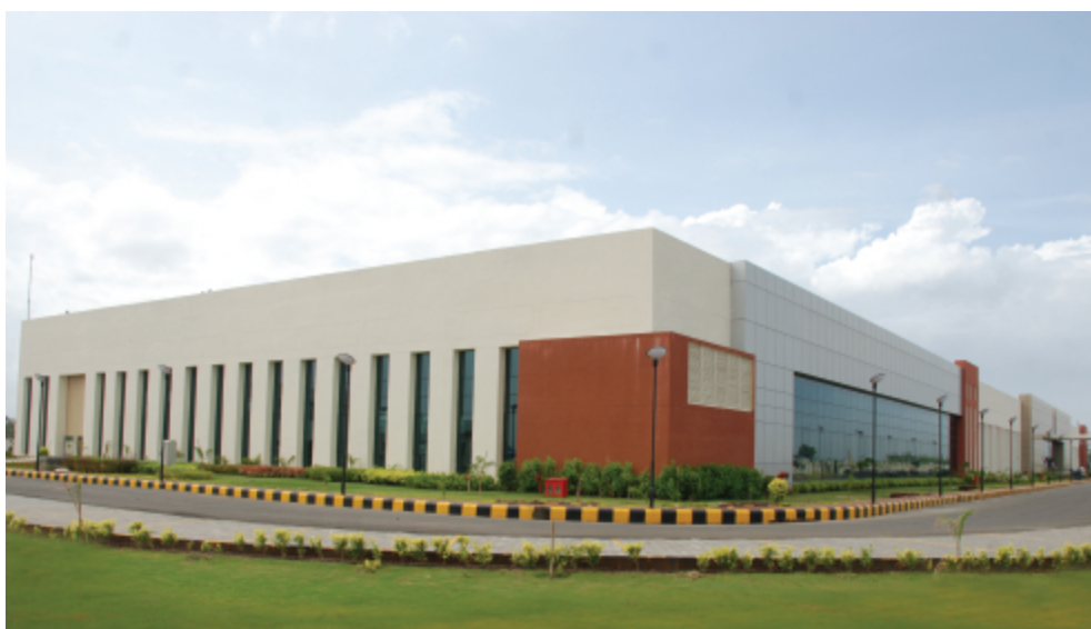
Switchgear Factory, Baroda
