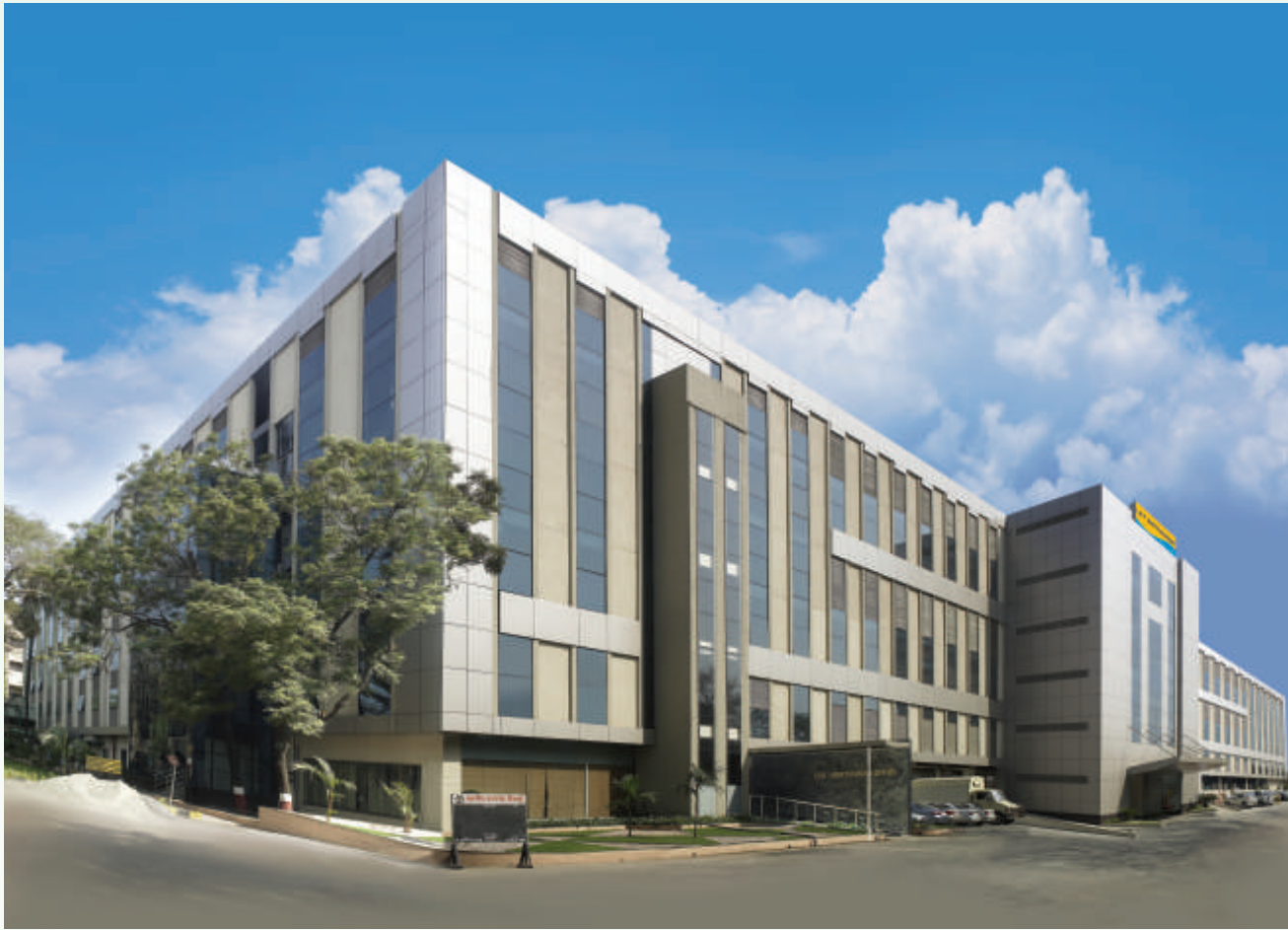
Switchgear Factory, Mumbai
