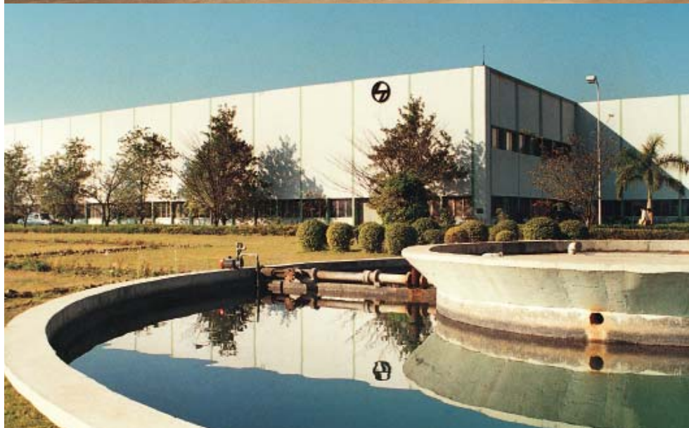
Switchgear Factory, Ahmednagar
