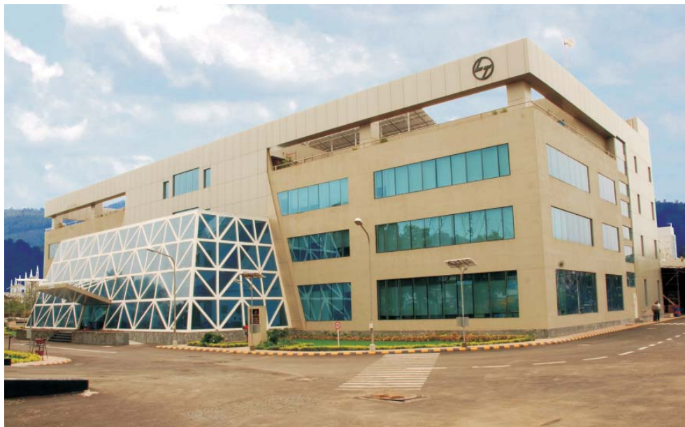
Switchgear Factory, Navi Mumbai
