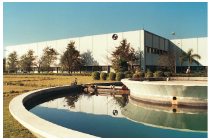
Switchgear Factory, Ahmednagar
