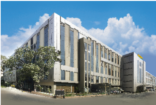
Switchgear Factory, Mumbai
